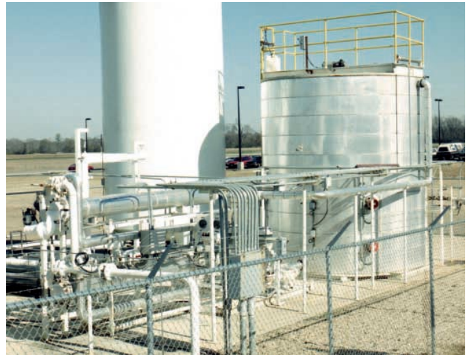
This complete nitrogen pressurization system for a McGill autoclave includes two liquid nitrogen tanks and a hot-water-heated nitrogen vaporizer.
